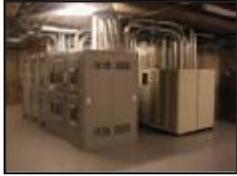
These industrial-grade devices, often called a UPS, are manufactured by PowerWare. They act like huge surge protectors, providing clean power to the entire facility. The UPS subsystem is tied into both the utility power and the back up diesel generator power
