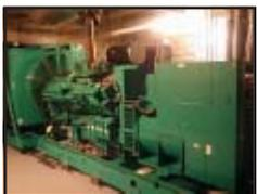
The 1,500 kilowatt diesel generator is one of the largest commercially available generators found in a managed hosting facility. The day fuel tank holds 100 gallons. A reserve tank (16 feet in diameter) provides an additional 6,000 gallons of fuel. Fully
